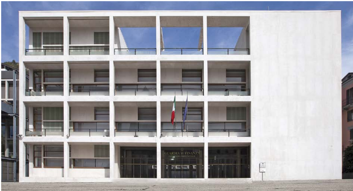
Fig. 1 Giuseppe Terragni, The Casa del Fascio, 1932-1936. Structure in reinforced concrete, finished in plaster and varieties of marble. Como.
