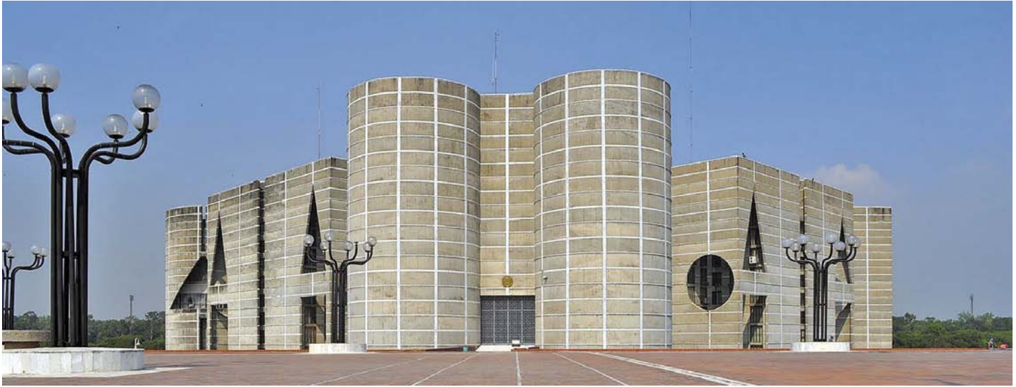
Fig. 3, 4 Louis Kahn, National Assembly Building, 1962-1973. Dacca (Bangladesh), general view and plan (below).
